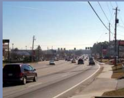
Five-Lane Roadway (no median)
